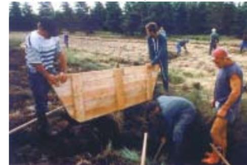
INSTALLATION D'UN BARRAGE SEUIL EN PLANCHES DE BOIS.
